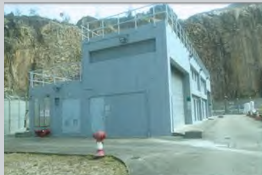
CCTV, Explosive Ordnance Disposal
